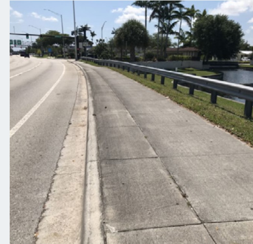
Minimal shade along Commercial Blvd.
