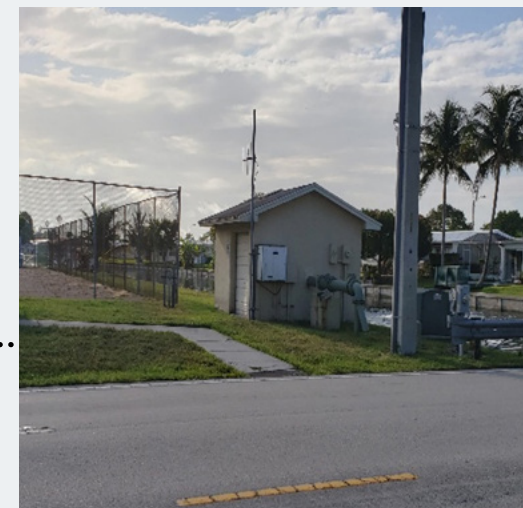
Sidewalk ends on NW 84th Terrace
