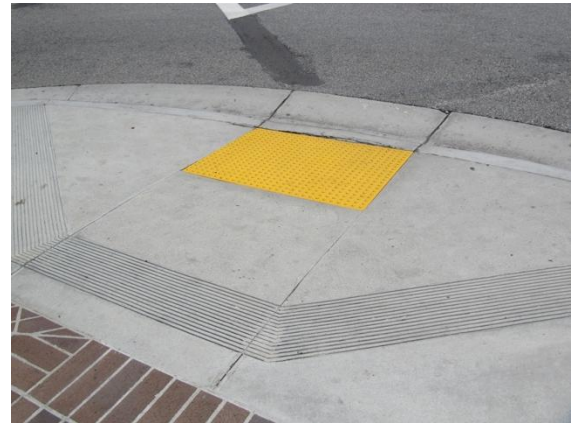
Required truncated domes (Credit: Ryan Snyder)
