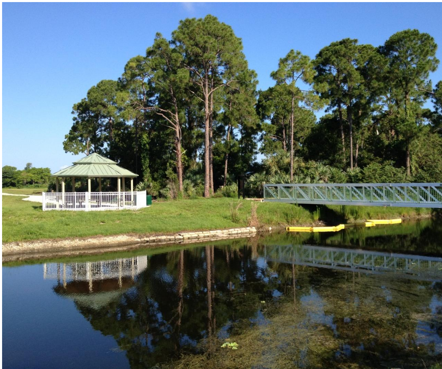
(Credit: Kimley-Horn and Associates, Inc.)
