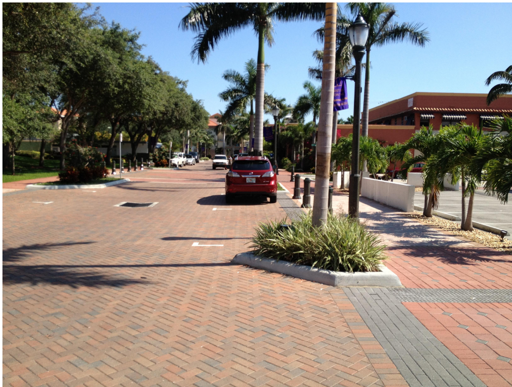
Landscaped curb islands, decorative pavers, and no centerline stripe help give this festival street a sense of place while calming traffic (Credit: Kimley-Horn and Associates, Inc.)
