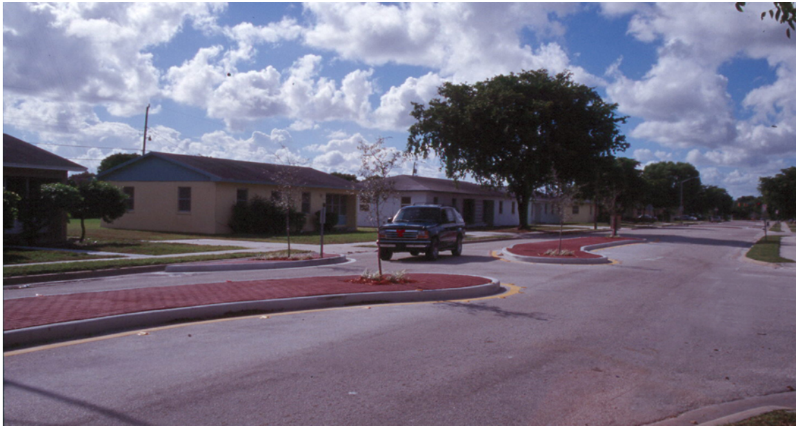
Impeller T-intersection (Credit: Ian Lockwood)
