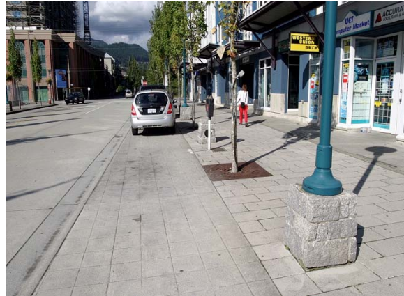
Valley gutter (Credit: Ian Lockwood)
