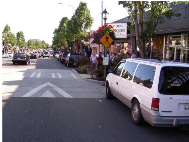
Periodic traffic calming measure: Raised crosswalk in Seattle, WA (Credit: Ryan Snyder)
