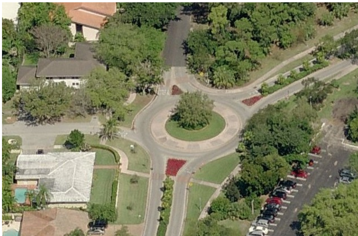
Roundabout with splitter islands for pedestrian crossings (Credit: Kimley-Horn and Associates, Inc.)
