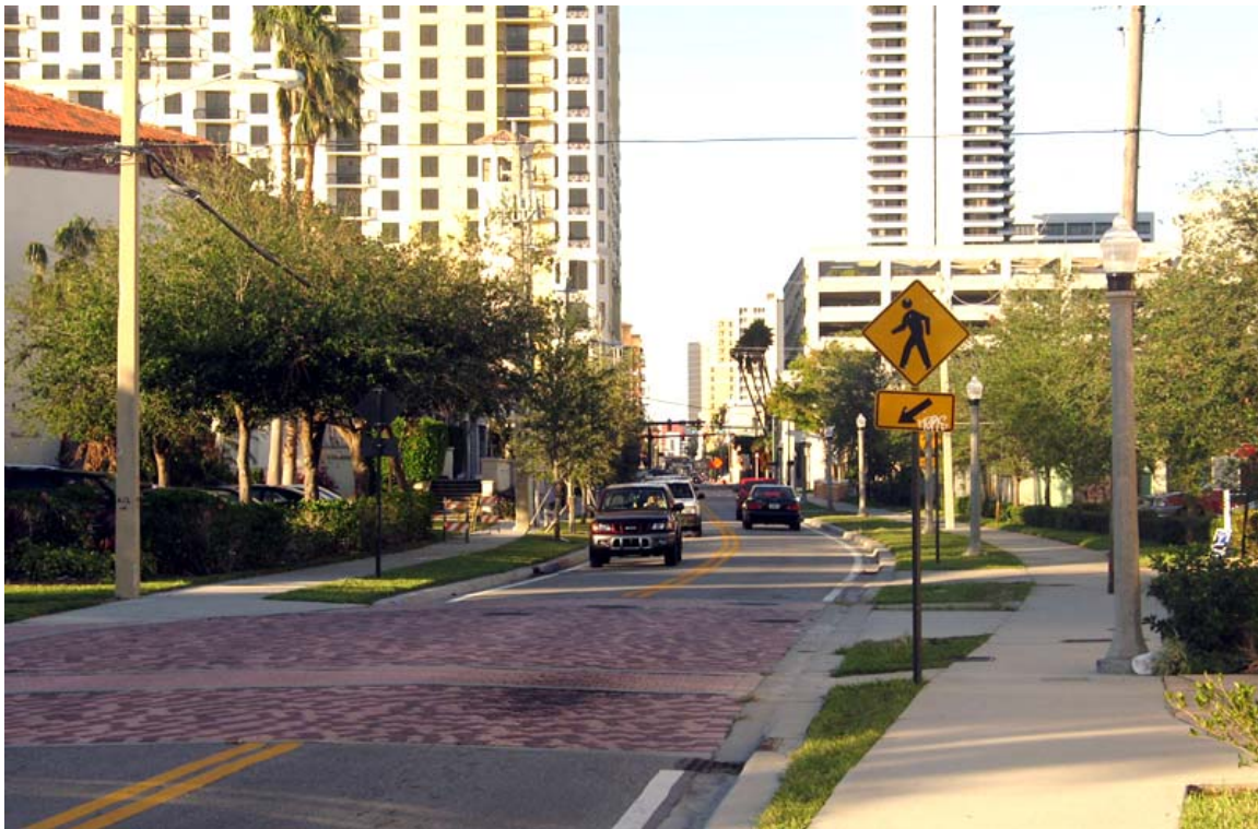
Raised crosswalk (Credit: Ian Lockwood)
