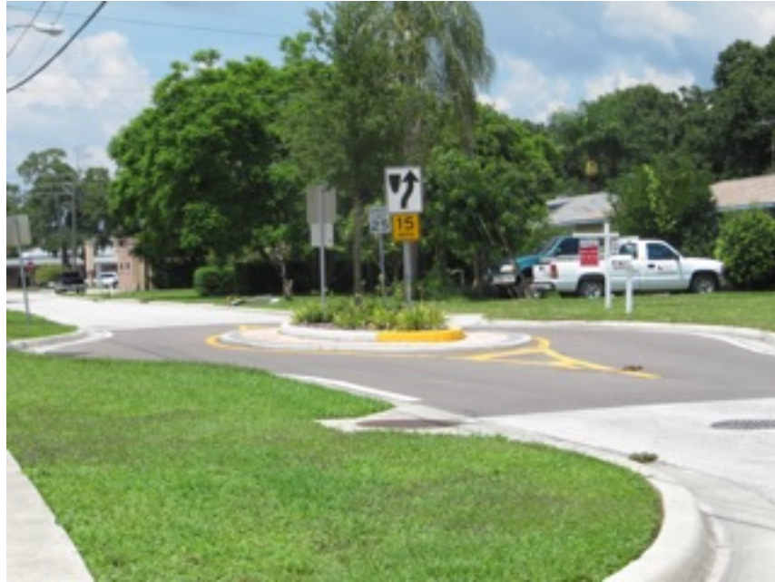
Oval median (Credit: Michael Wallwork)
