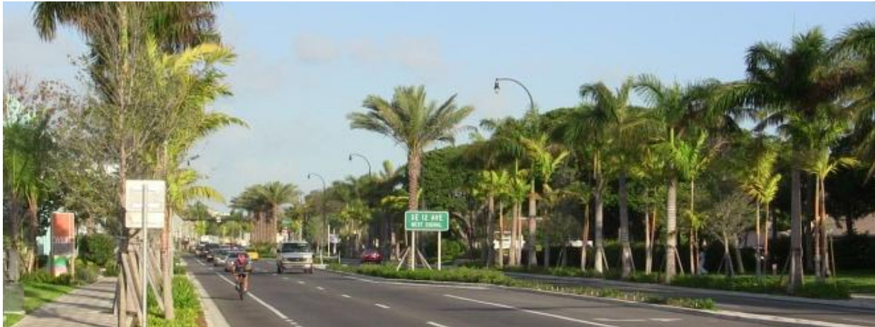
Hillsboro Boulevard bike lane and streetscaping (Credit: City of Deerfield Beach)
