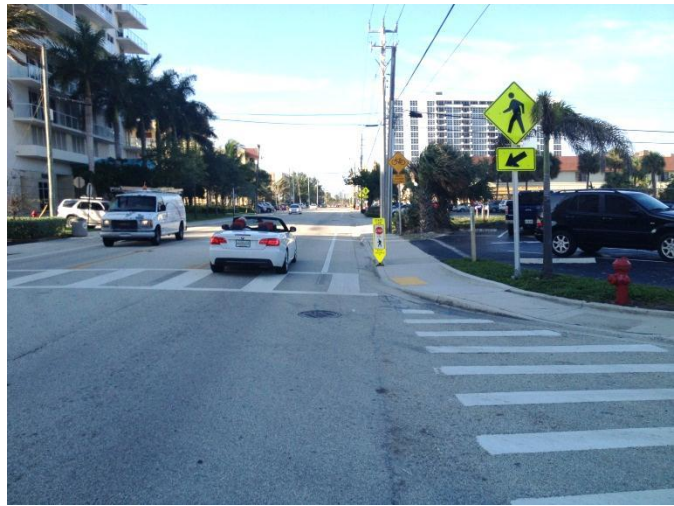
Pedestrian crossing at an uncontrolled intersection (Credit: Kimley-Horn and Associates, Inc.)
