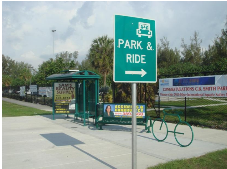
Transit shelter with bench and bicycle parking adjacent to park-and-ride lot, Pembroke Pines
