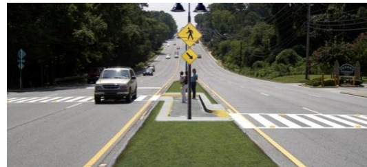
Staggered median crossing (Credit: Marcel Schmaedick)
