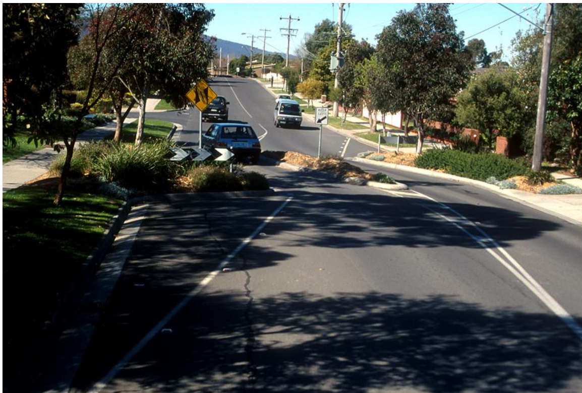
Two-lane chicane (Credit: Michael Wallwork)
