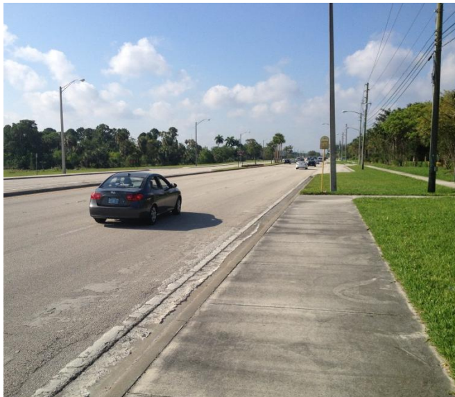
Sidewalk on a suburban boulevard in Broward County near a bus stop (Credit: Kimley-Horn and Associates, Inc.)
