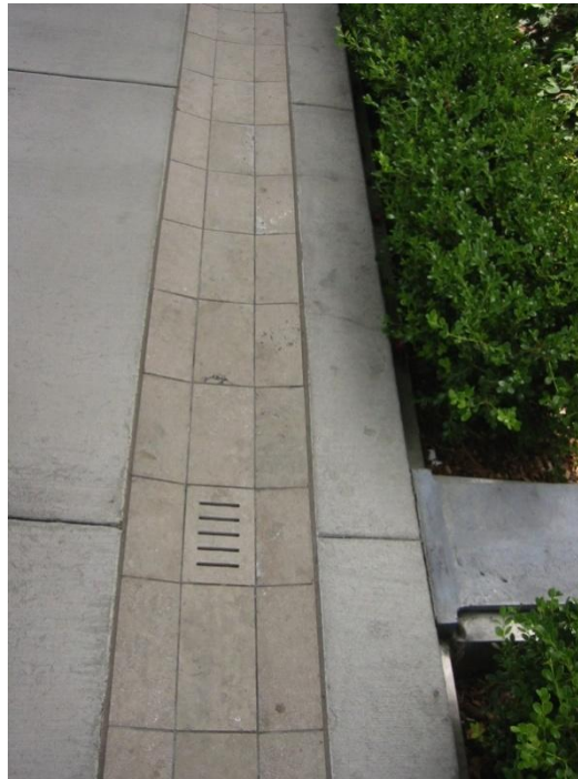
Constructed swale with drain (Credit: Stephanie Landregan)
