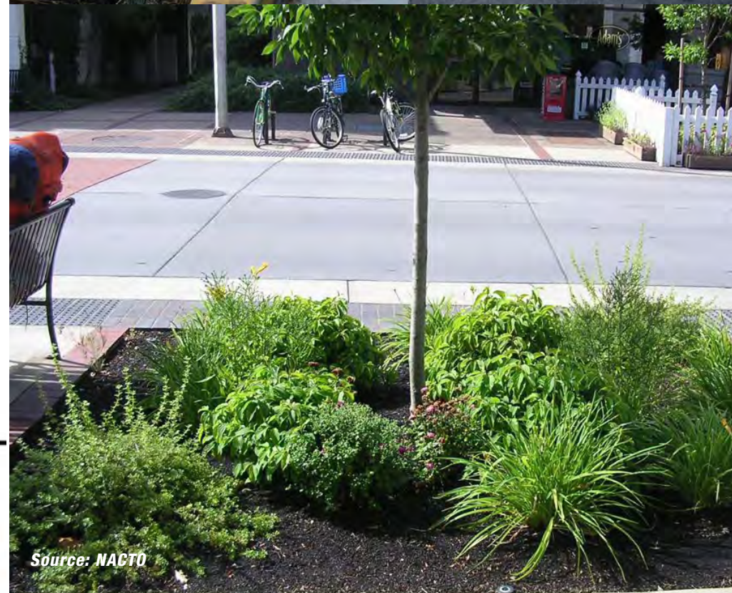
Bioswales installed at a mid-block crossing
