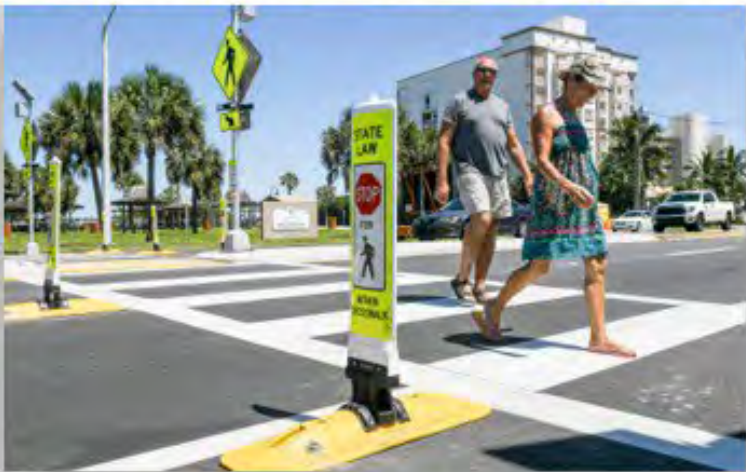
Rectangular Rapid Flashing Beacon
