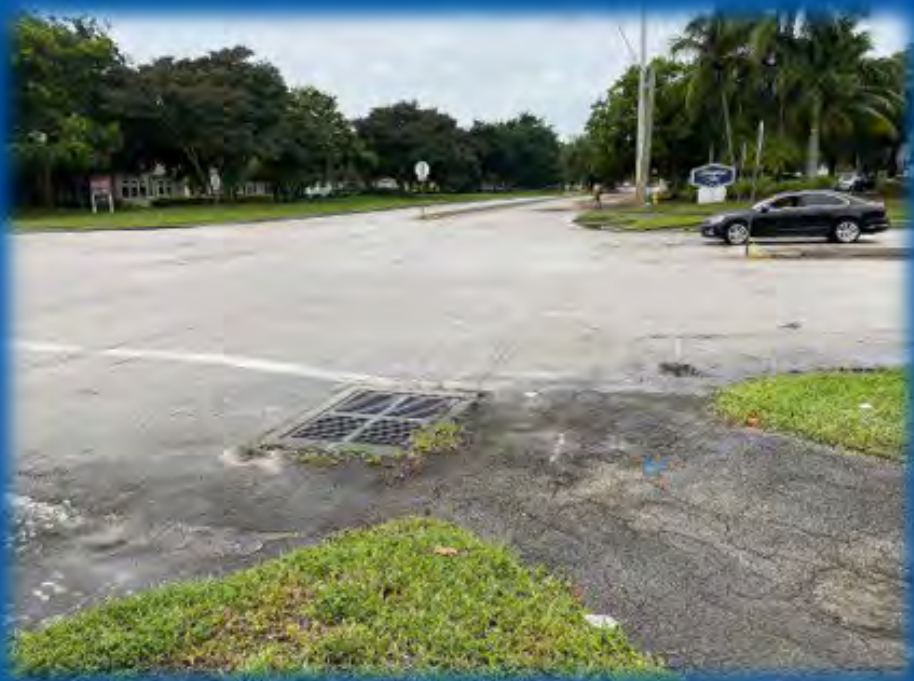
Intersection of SW 6 th St and SW 78 th Av @ NE corner, looking west. No crosswalks, no pedestrian scale lighting, drainage located within crosswalk area
