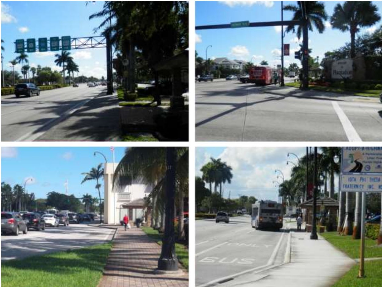
Figure 3-44: Broward Boulevard Field Review Photos
