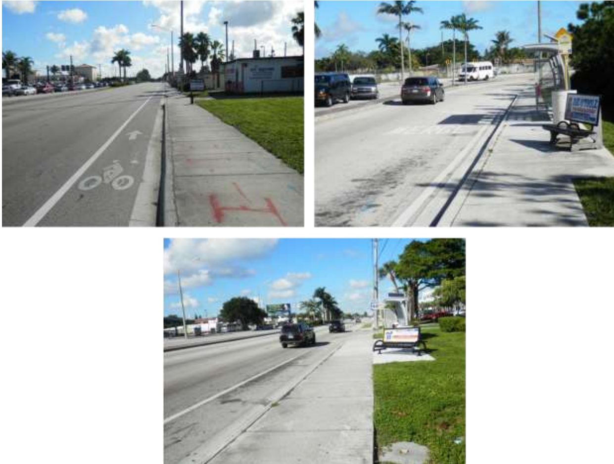
Figure 3-40: Riverland Road Field Review Photos
