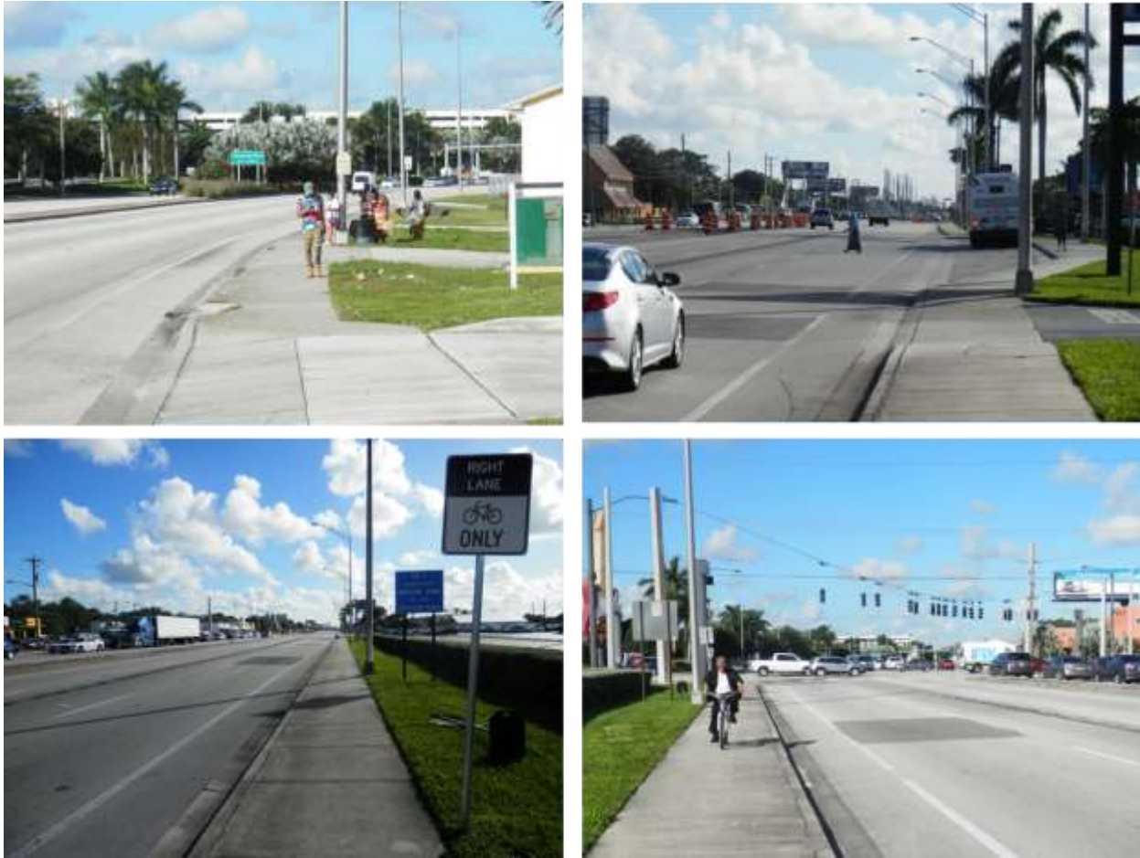
Figure 3-38: Stirling Road Field Review Photos
