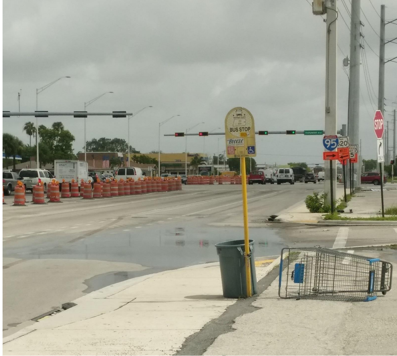
Hollywood Blvd and SR 7 - Northbound Near Side
