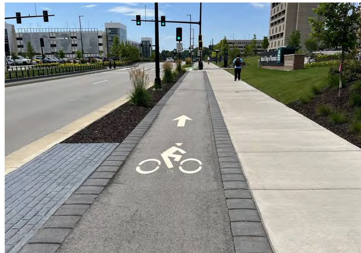
Raised Bike Lane
