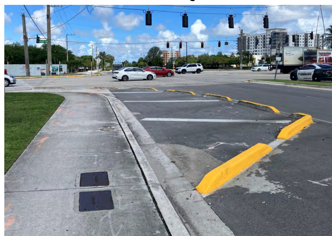
Curb Extension – Quick Build
