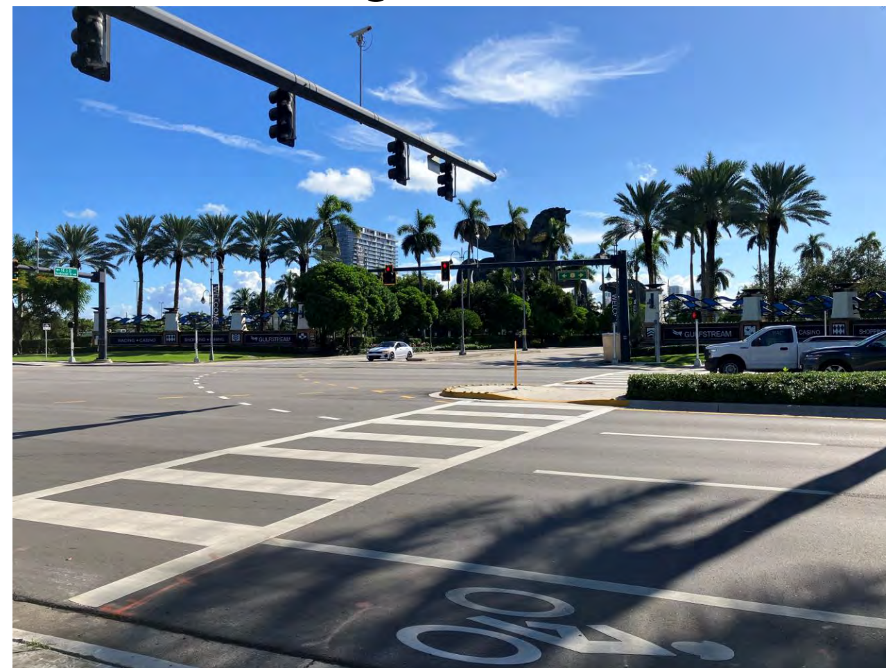
Median Refuge Island
