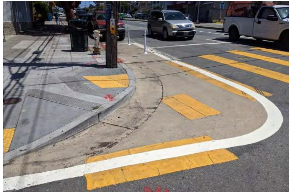
Curb Extension – Quick Build
