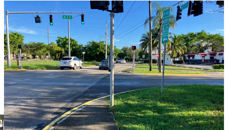
(View from SE corner) No curb ramp to cross the east leg; despite pedestrian signal, no crosswalk over north leg
