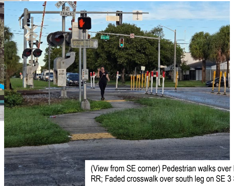
(View from SE corner) No curb ramp to cross the east leg; despite pedestrian signal, no crosswalk over north leg
