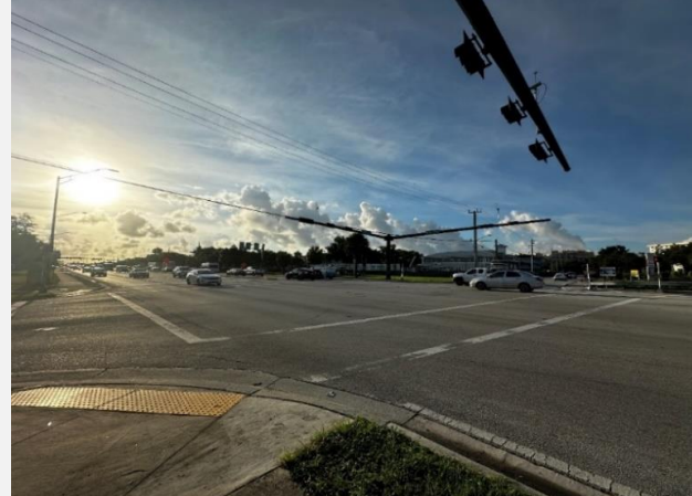
Lack of high-emphasis crosswalk on Atlantic Blvd
