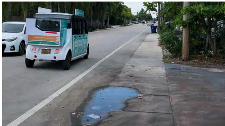
East sidewalk is at grade; ponding on sidewalk
