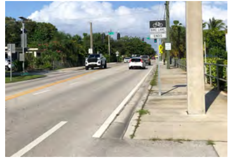
Bike Lane and WME School Zone end west of intersection; SW sidewalk widens to shared use path; No signage telling bicyclists to ride on roadway or sidewalks; Numerous sidewalk obstructions
