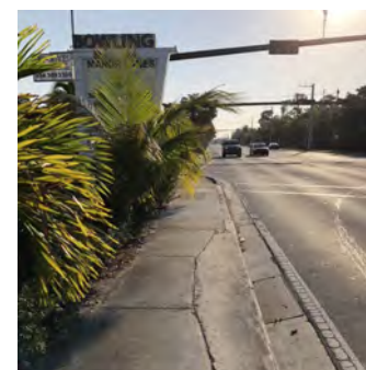
Overgrown landscaping in front of Bowling Alley obstructing sidewalk
