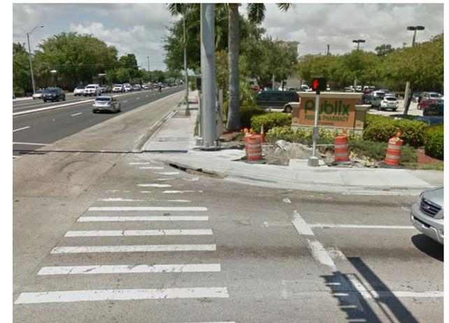
The drainage inlet on the northwest corner of NE 15th Avenue blocks the ramp.
