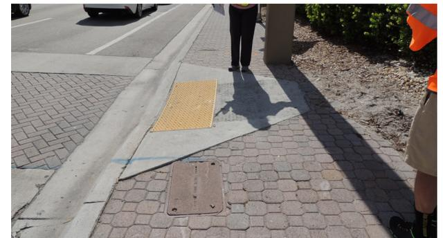
The sidewalk does not provide a level surface behind the ramp as required by ADA.
