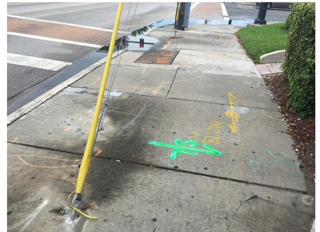
Support wires cause a tripping hazard in the sidewalk.
