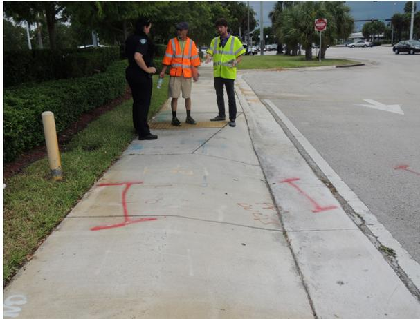
Improperly placed detectable warning surfaces and unnecessary ramp.
