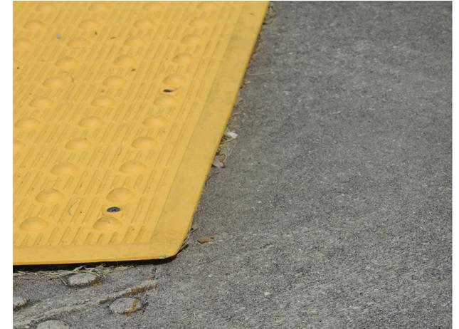
Improperly secured detectable warning surfaces.
