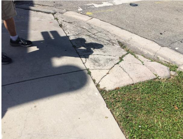
Lack of detectable warning surfaces and broken sidewalk.
