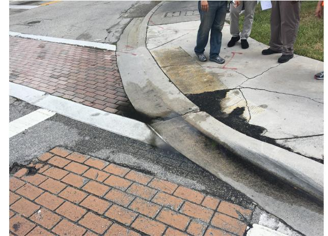
Cracked sidewalk and missing detectable warning surfaces on ramp. Crosswalks do not line up properly.
