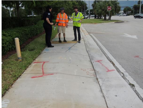
Improperly placed detectable warning surfaces and unnecessary ramp.
