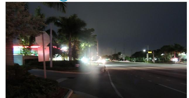
Lighting is poor outside of signalized intersections and present only on one side of the street.
