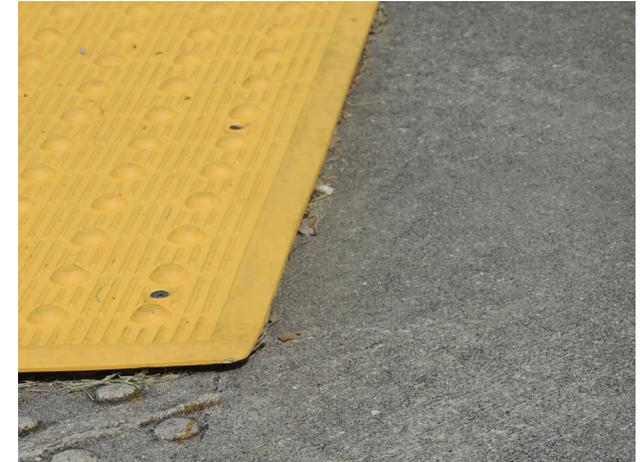
Improperly secured detectable warning surfaces.
