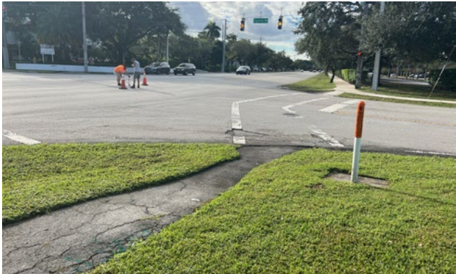
Cypress Rd and NW 70th Av intersection (west view); Cypress Rd widens to include striped median. Curbs and crosswalks are in poor condition.
