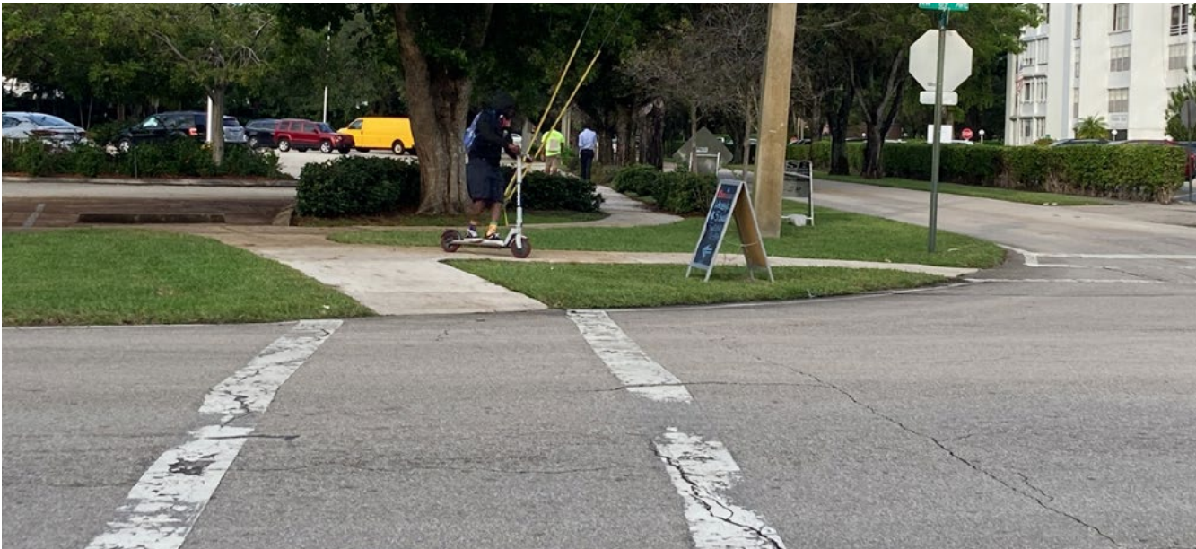
SE corner of Cypress Rd and NW 69th Av (west view); Faded crosswalks and adjacent sidewalk veers into parking lot.
