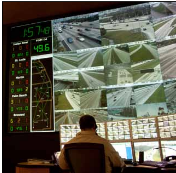
Monitoring traffic flow at the Broward County/FDOT Regional Transportation Management Center
