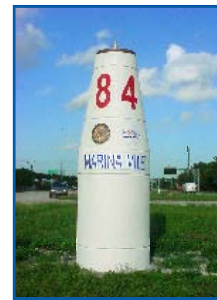
Buoy construction completed - September 2005.
