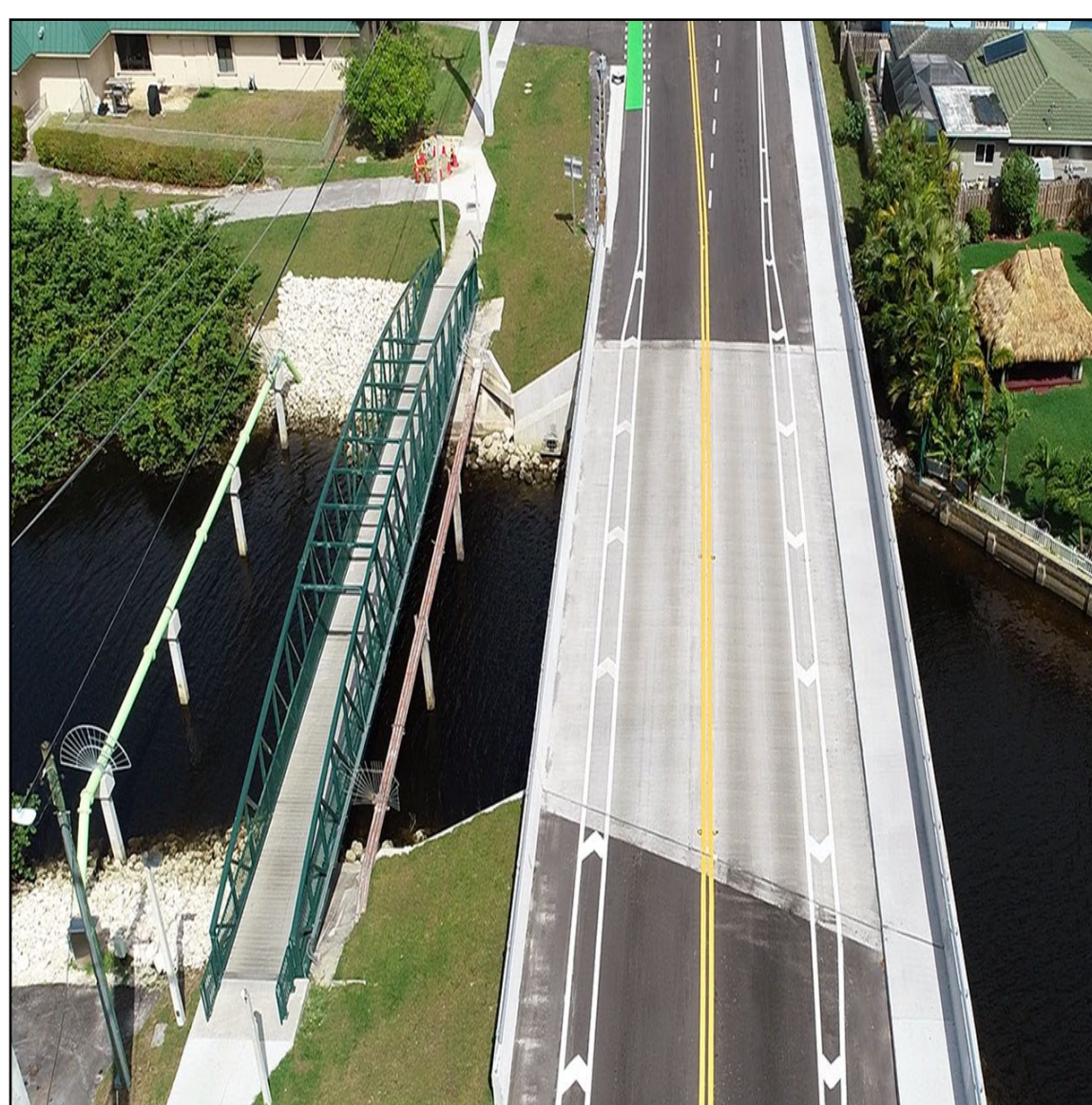
Pedestrian Bridge Over Canal
