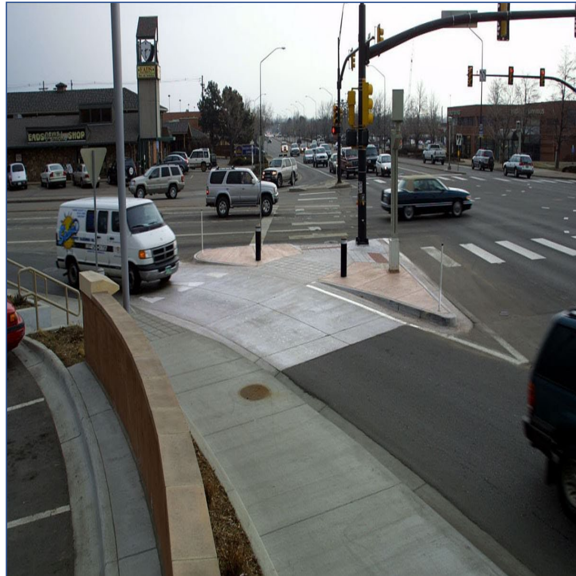
Right-turn Raised Median (Pork Chop) with Raised Crosswalk
