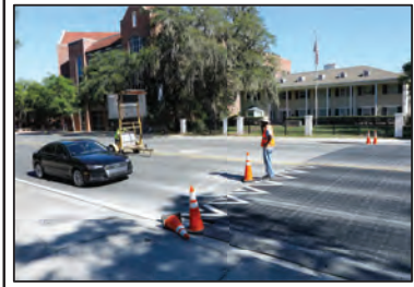
Quick Build Raised Crosswalk
