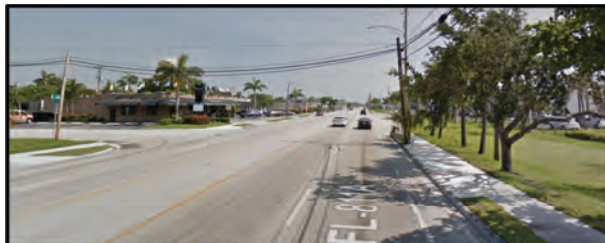
Before / After: Center Lane Median on Andrews Av, north of Oakland Park Blvd
