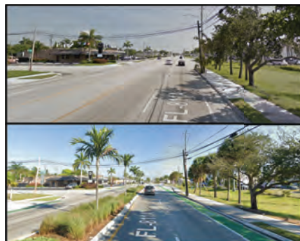
Before / After: Center Lane Median on Andrews Av, north of Oakland Park Blvd
