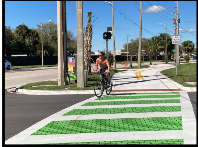
High Visibility Pavement Markings
