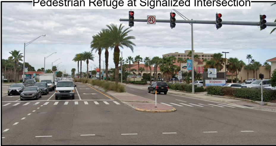
Pedestrian Refuge at Signalized Intersection
