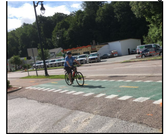
Shared Use Path Conflict Markings
