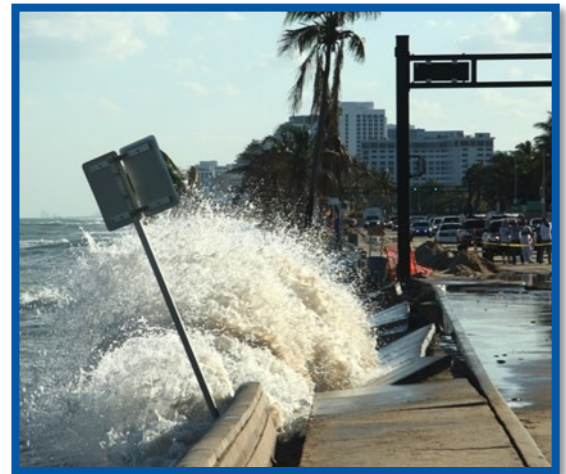
Superstorm Sandy washes out A1A in Fort Lauderdale. (Photo by Art Seitz)
