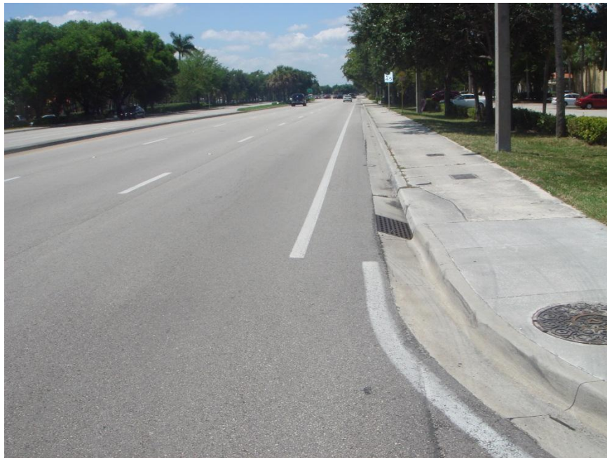
Undesignated lane. Note the corner radius striping, which allows bicycles to enter the undesignated lane. (Credit: Kimley-Horn and Associates, Inc.)
