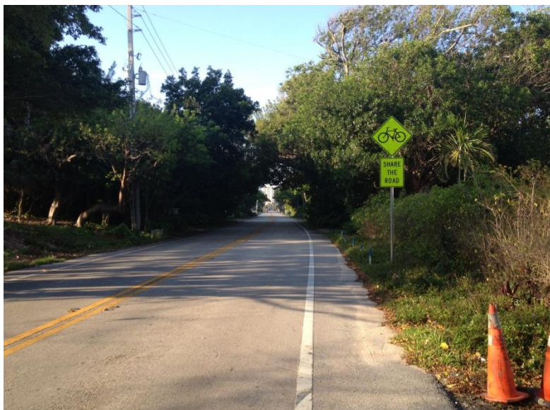
Paved shoulder with Share-the-Road sign assembly (Credit: Kimley-Horn and Associates, Inc.)
