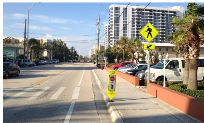
Uncontrolled mid-block pedestrian crossing (Credit: Kimley-Horn and Associates, Inc.)
