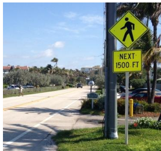
Advance pedestrian warning sign with distance plaque (Credit: Kimley-Horn and Associates, Inc.)
