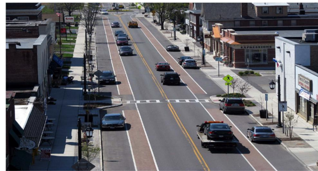
Parking assist lane (Credit: Michael Wallwork)
