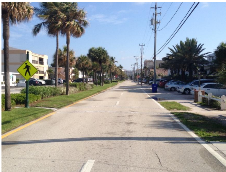
Avenue example (Credit: Kimley-Horn and Associates, Inc.)
