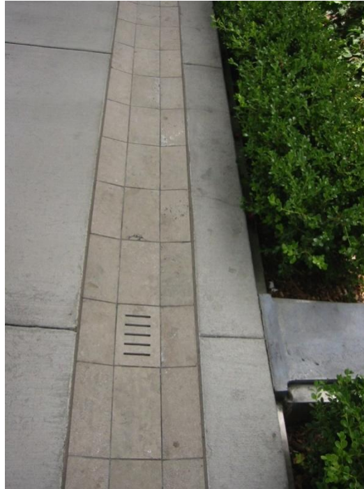
Constructed swale with drain (Credit: Stephanie Landregan)
