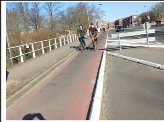
Worn out paint on a temporary painted bike lane in Delft
