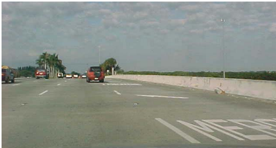
Exhibit 19. Concrete barrier wall on westbound I-75 bridge deck
