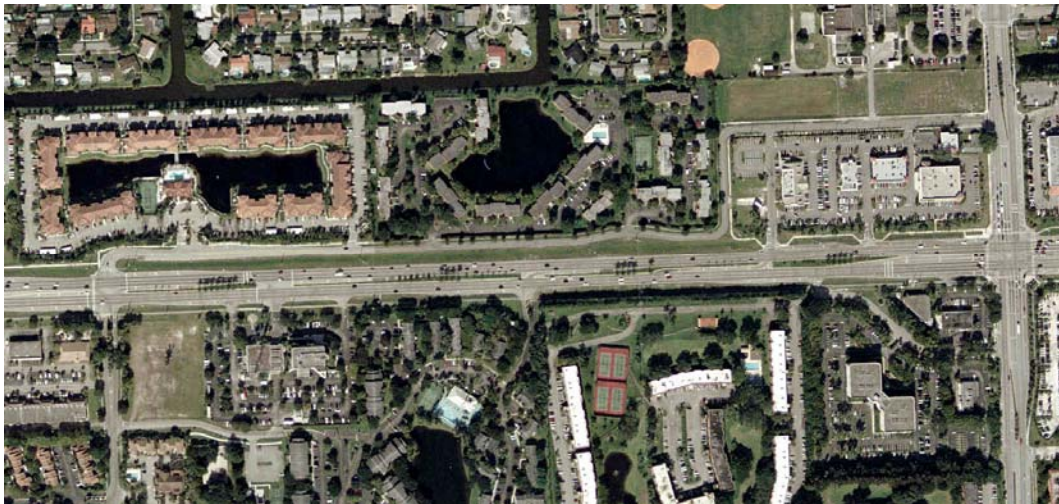
Exhibit 21. Aerial photograph showing sidewalk discontinuity on north side of roadway
