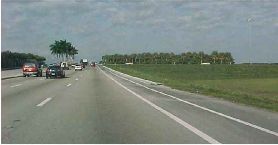
Exhibit 18. Westbound approach to the I-75 bridge
