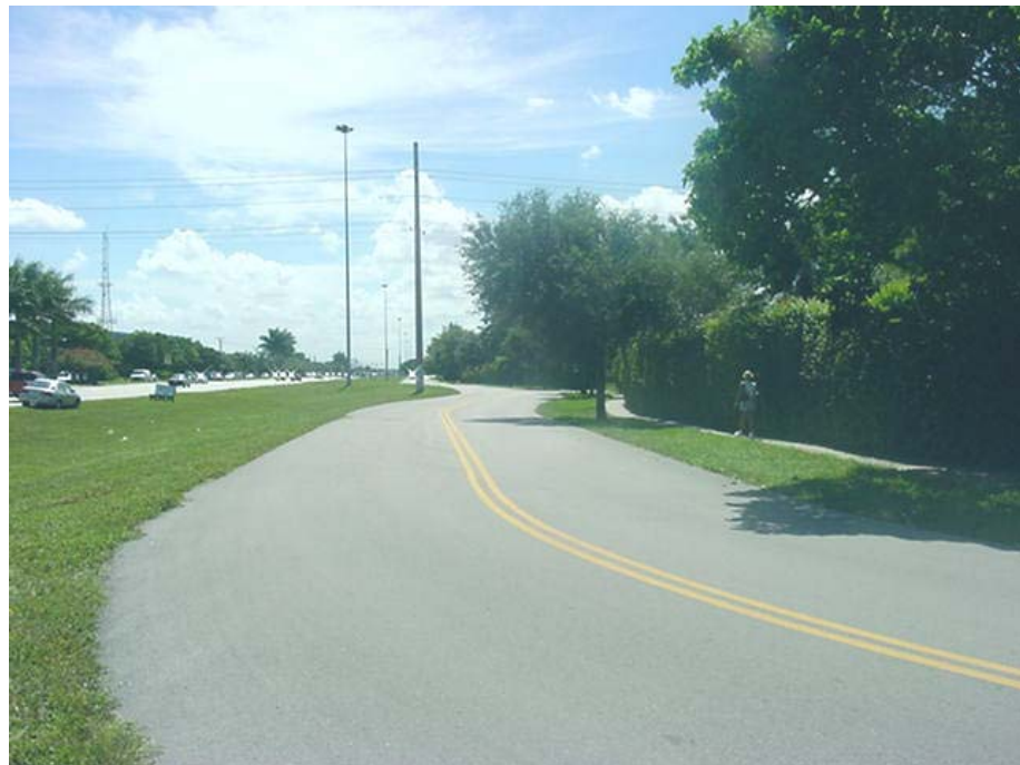
Exhibit 2. Sidewalk discontinuity 900 feet west of Douglas Road (facing WB)
