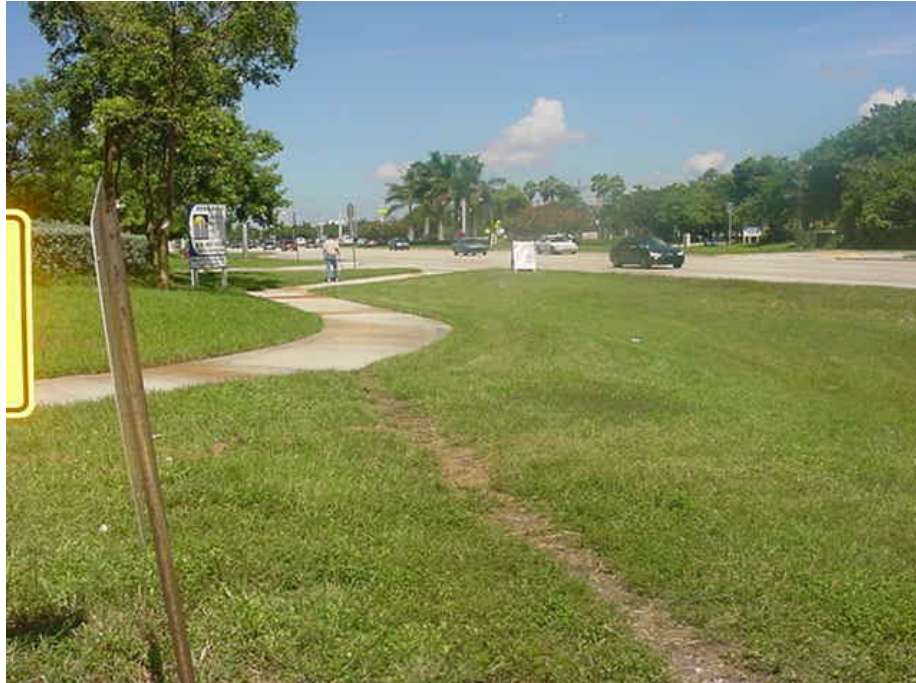
Exhibit 1. Sidewalk discontinuity 900 feet west of Douglas Road (facing EB)
