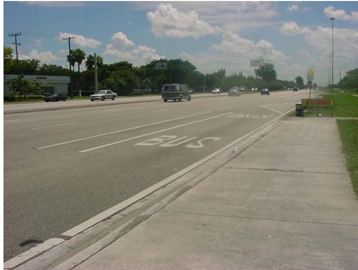
Exhibit 6. Bike lane along westbound Pines Boulevard west of Douglas Road
