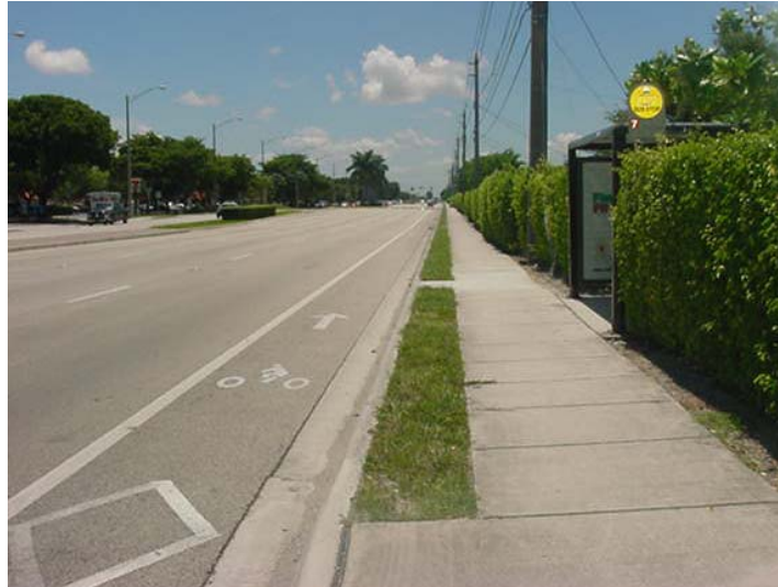
Exhibit 25. Existing bike lane along Hollywood Boulevard in the vicinity of 68 th Avenue
