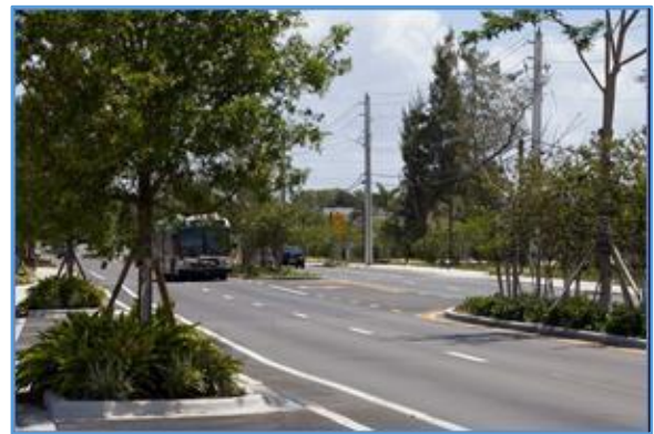
Figure 5 Hammondville Road Existing Complete Streets improvements (East of proposed project)
