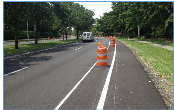
Figure 2 Buffered Bicycle Lane Currently Under Construction
