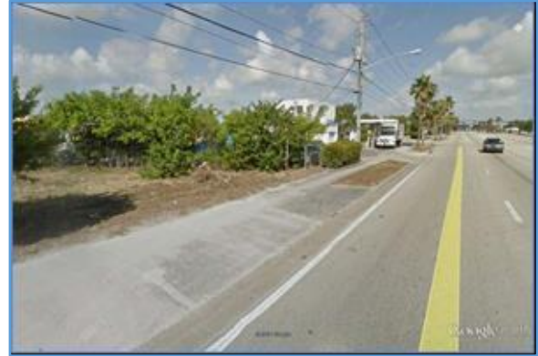
Figure 4 Hammondville Road (Existing)
