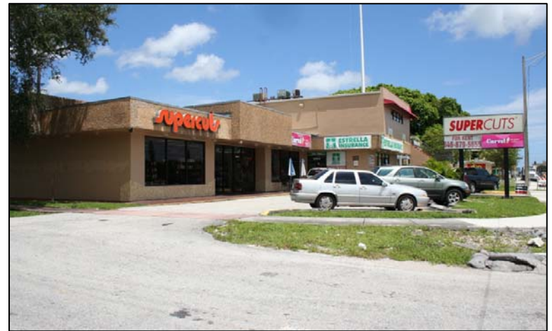
Figure 5-3: Example of existing conditions in Transitional Segment – Hollywood Blvd and SR 7
