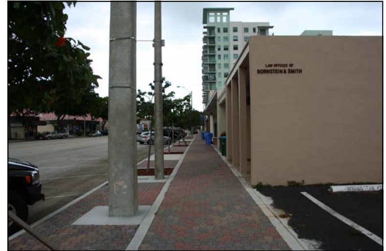
Figure 4-3: Example of a sidewalk along Hollywood Boulevard
