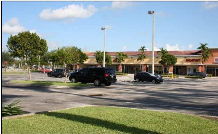
Figure 5-4: Example of existing conditions within Suburban segment – Pines Blvd and Dykes Rd
