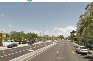
Frequent turn lanes limit space, allowing only for concrete curb medians.
