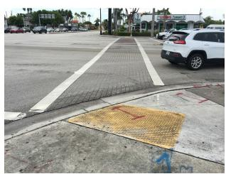
Ramp does not meet ADA requirements; detectable warning surfaces are cracked/inadequate,
