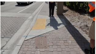
The sidewalk does not provide a level surface behind the ramp as required by ADA.
