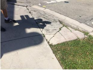
Lack of detectable warning surfaces and broken sidewalk.
