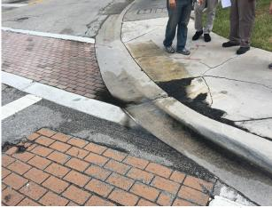
Cracked sidewalk and missing detectable warning surfaces on ramp. Crosswalks do not line up properly.
