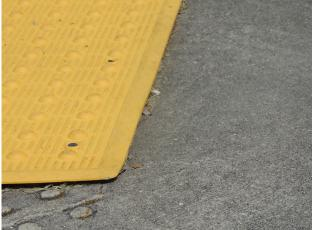
Improperly secured detectable warning surfaces.
