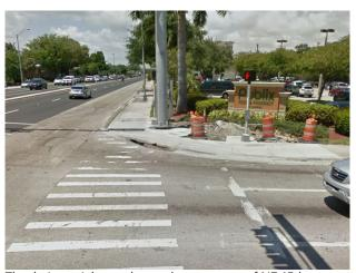
The drainage inlet on the northwest corner of NE 15th Avenue blocks the ramp.
