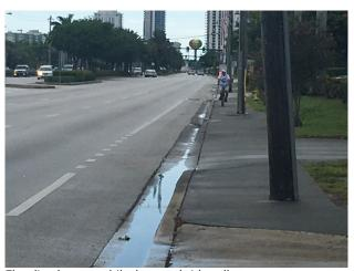
Flooding between bike lane and sidewalk.
