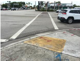
Ramp does not meet ADA requirements; detectable warning surfaces are cracked/inadequate,
