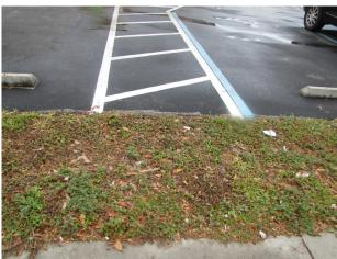
No accessible sidewalk connection between sidewalk and parking lot.
