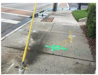
Support wires cause a tripping hazard in the sidewalk.
