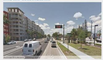
The corridor has a three lanes in each direction. It has intermittent right- and left-turn lanes. It also has median with intermittent landscaping, cobra style vehicular lighting, and dynamic message signs. The corridor has 5' - 7' sidewalks and no marked bike lanes or paved shoulders. The posted speed is 35 MPH. The land uses are redeveloping; new buildings front the street while older buildings and shopping centers are set behind large surface parking lots.
