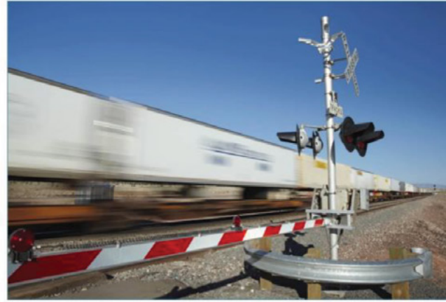
In Florida, the project will increase safety at 21 grade crossings along the state's East Coast Rail Corridor.
