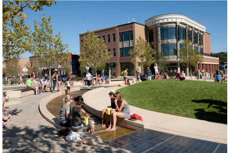
Normal, Illinois used a TIGER grant to build a new multimodal transportation hub and revitalize the Uptown core (pictured), which spurred millions in new economic development. Photo courtesy of Scott Shigley. Read more: http://t4america.org/maps-tools/local-successes/normal
